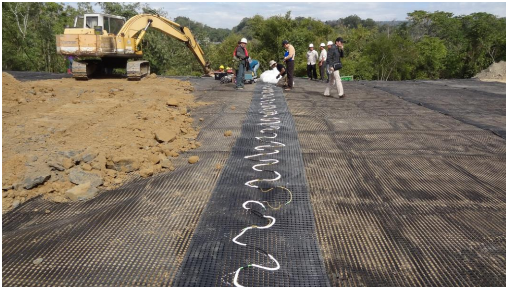
Figure 5. Unrolling of the instrumented geogrid.
